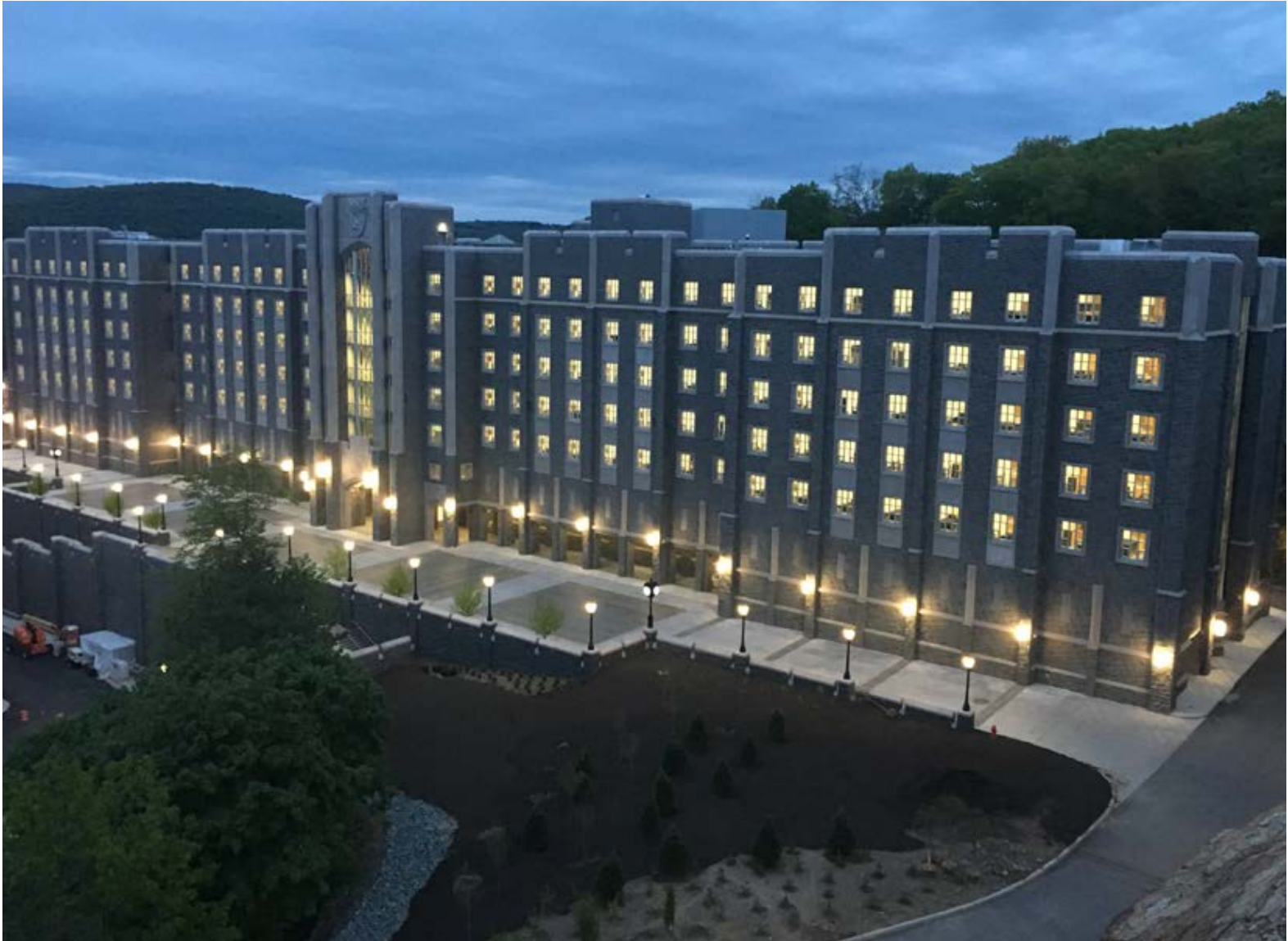
Radiant heating and cooling systems, solar thermal panels, day-lighting technology, and the use of energy efficient lighting and controls all contribute to the LEED Silver status of the new General Benjamin O. Davis Jr. Barracks at West Point. PHOTOS COURTESY WALSH CONSTRUCTION AND ACADEMY ENERGY GROUP
